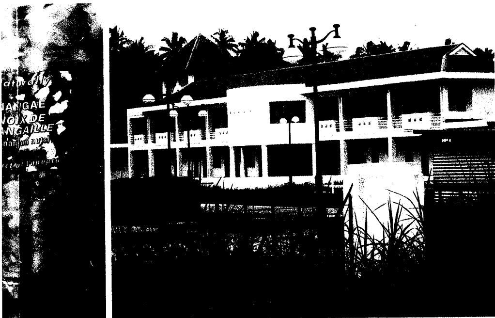
Built by the Chinese...Vanuatu's new agricultural school.
